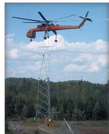
Figure 6: Sky Crane Lifting Communication Tower
